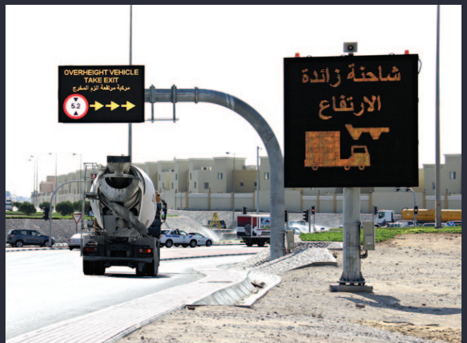
The Duhail Interchange Over-height Vehicle Detection System
